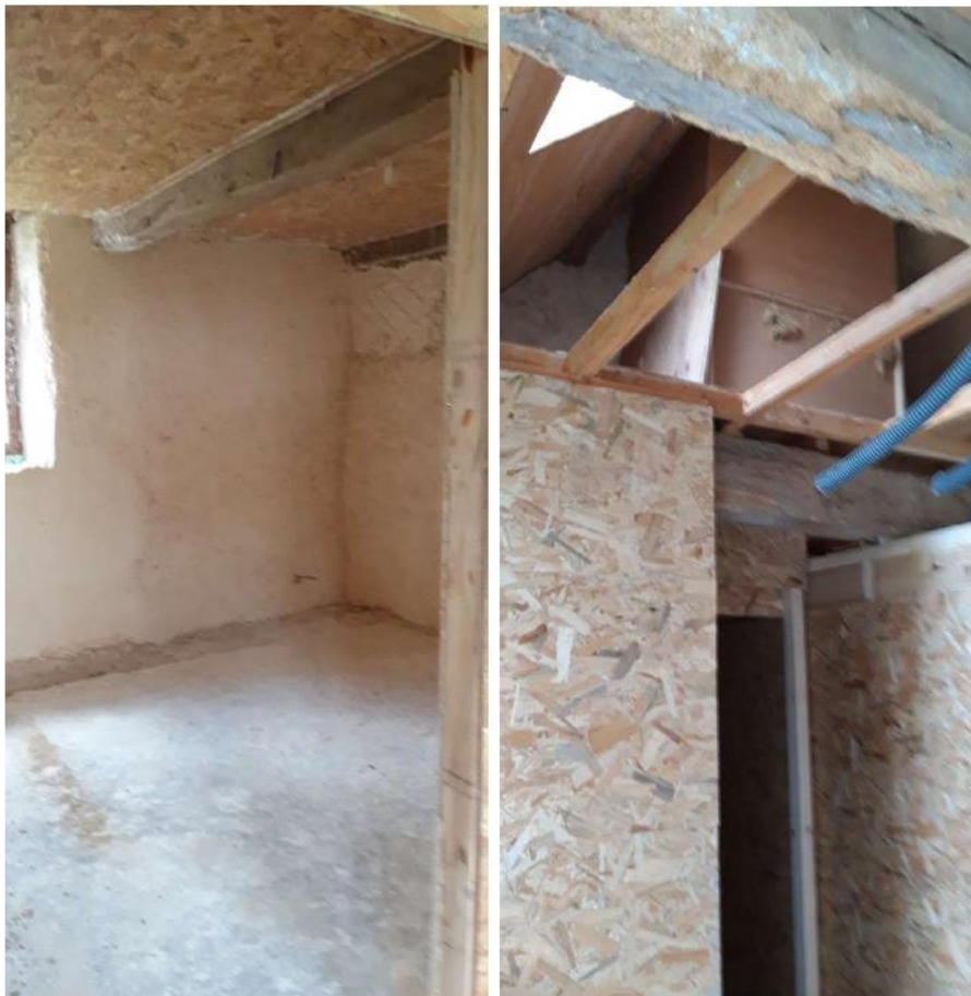
Hemp filler on external walls for humidity regulation and thermic correction
