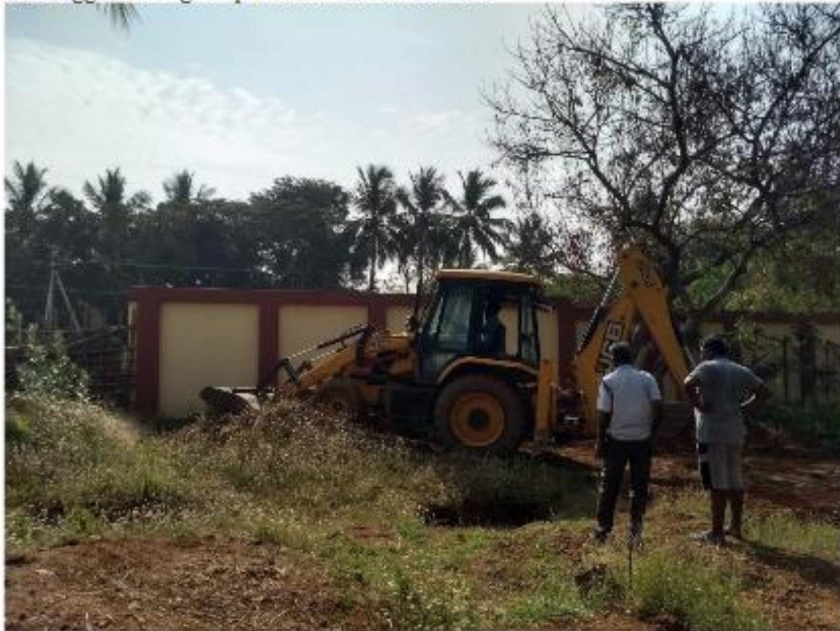
JCB digger closing the previous foundation holes
